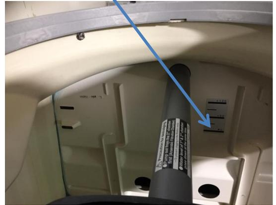
Please note: To assure tank water tightness, please check in 24 hours to be sure that the water level has not dropped. Please contact your distributor or Fuji Clean USA if water level has dropped.
