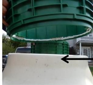
Apply sealant for watertight seal.
