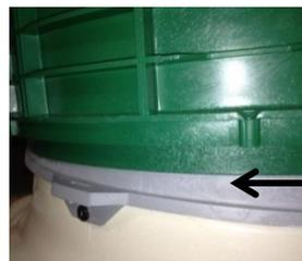
Use sealant that meets ASTM C990-96 Standard here.
