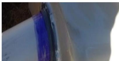
Apply primer and cement to 4" Sched. 40 PVC inlet and outlet pipe sections
